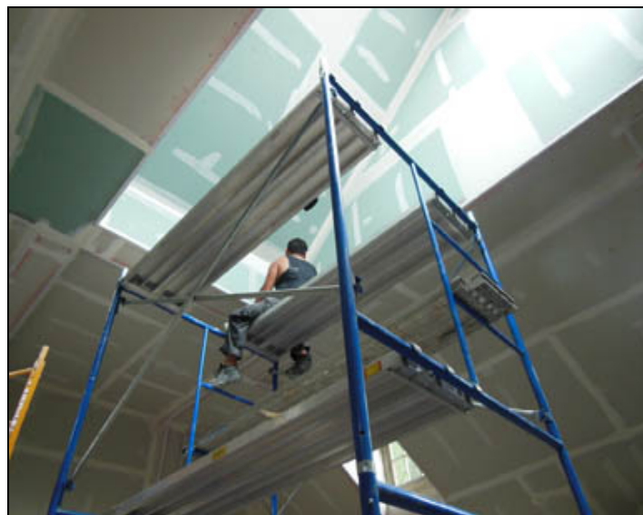
Interior of the Shiekman Studio under renovation.
